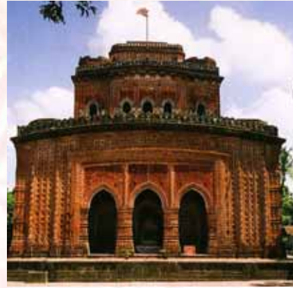
Kantiji Temple constructed with bricks and terracotta.
